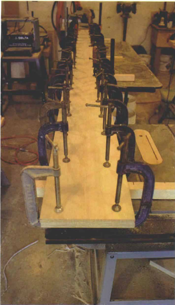
Laminated stringers won't shrink or warp. Two layers of \frac{3}{4} in. plywood are glued together for stringer stock that will remain stable and true for the life of the stair.
