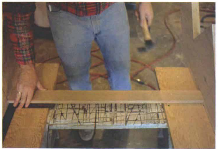
Witness marks help align the stringers in the jig. Lines called witness marks are made with the stringers laid side by side. Then a square and a straightedge align one stringer perfectly with the other.
