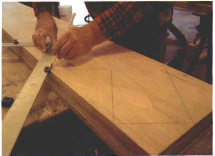
Each tread/riser layout is duplicated exactly. Stair gauges clamped to the edge of a framing square allow the layout to be repeated precisely for each step.
