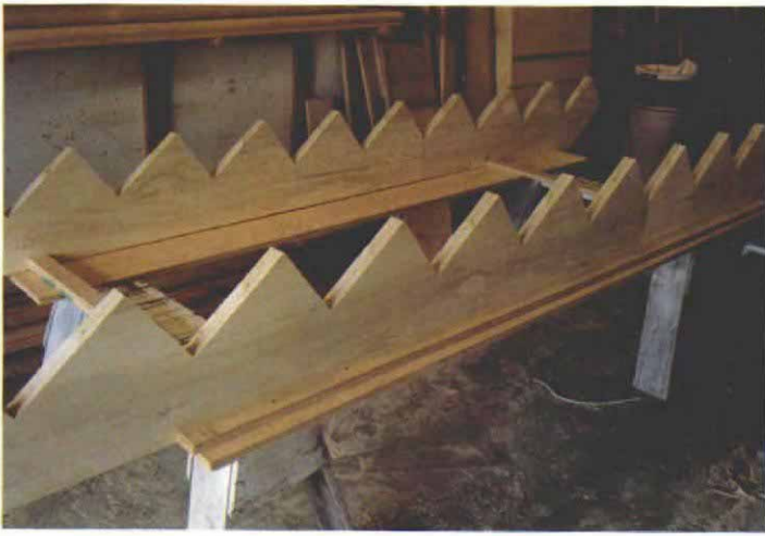
Assembly jig holds the stringers parallel and square. A simple jig made from strips of plywood holds the stringers at the proper width while the author is attaching treads and risers.
